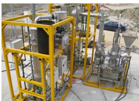
Picture 4: Another general view of the demonstration gasification / vitrification unit
